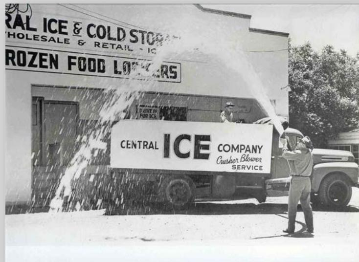
*Hugo Miller of Western Precooling demonstrates the first mobile block ice crusher and top-icing unit. Bob Kasmire of the Mann Lab was the key extension researcher in developing knowledge and application technology to support postharvest quality management of 'iceberg' lettuce during transportation and distribution. Digital image kindly provided by Craig Miller.*
