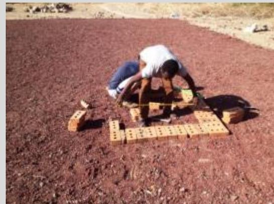
Constructing 100 kg capacity of Zero Energy Cooling Chamber (ZECC) from bricks and river sand at Samara Agricultural Research Center Compound of Ethiopia, for fruits and vegetables storage. ZECC is well known for reducing physiological loss in weight and decay loss in fruits and vegetables by lowering the temperature and increasing the relative humidity as compared to ambient conditions.
