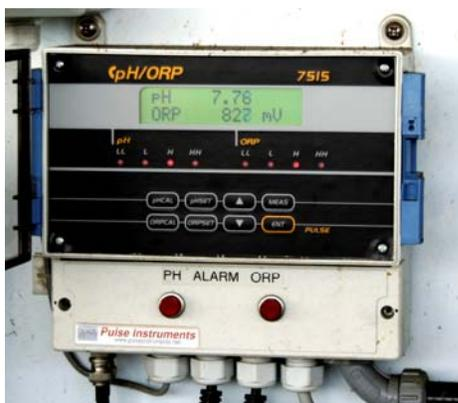
Fig. 5. Automated system monitoring the oxidation-reduction potential (ORP) and the pH of the water. ORP measurement is the most effective and direct way to monitor wash water sanitation activity.
